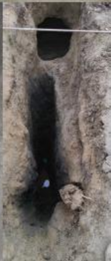
Several potholes required due to inaccuracy of miss dig staking
