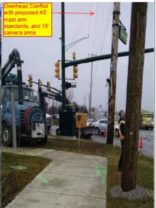
Several potholes required due to inaccuracy of miss dig staking
